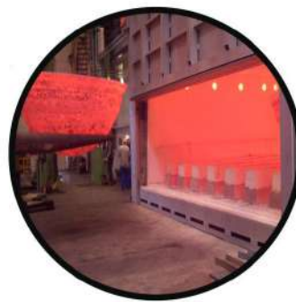
Industrial Furnace & Ovens
